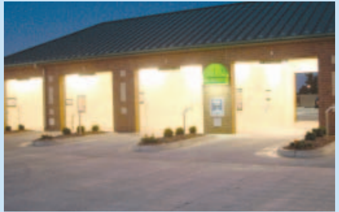
Lighting is very important. Customers will not wash in a dark location at night.
